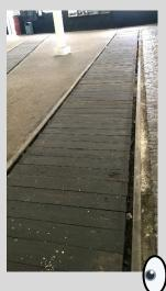
Look between the rails and you will see wooden boards that cover the maintenance pits. The pits are used by people mending the Locomotives so that they can get underneath to fix them.
