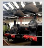
There are also smoke hoods. The hoods are over the place where a locomotive's funnel would be, to direct the smoke up and out.
