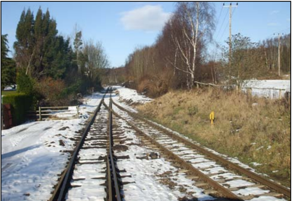
Looking North, the present running line on the old springwell colliery branch formation is on the left. Earth works and levelling for the new parallel siding are almost complete. The right hand turnout will be inserted into the plain panel of track at the 149 3/4 mile post.
